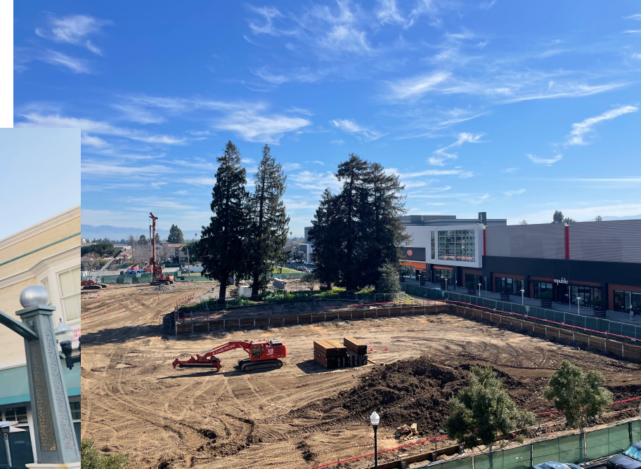
Finishing CityLine Sunnyvale Housing/Office/ Retail Construction
